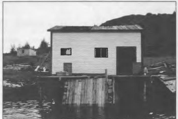
When work commenced, a new crib was constructed for the store and a new foundation was built. The store exterior received new clapboard and was painted, while the roof was repaired and covered in rubberoid. A new wharf was built to replace an earlier one that had been destroyed. Mr. Kippenhuck is proud of his family's long history with the site and was anxious to "restore the complete site to what it previously was before the closure of the cod fishery."
