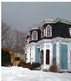
Excavator waits outside Quinnipiac
