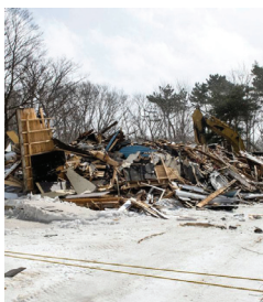
Moments after demolition
