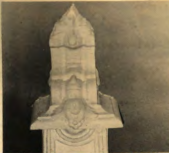
A detail from the hall moulding - one of the features that add interest to many of the older homes in the downtown.
