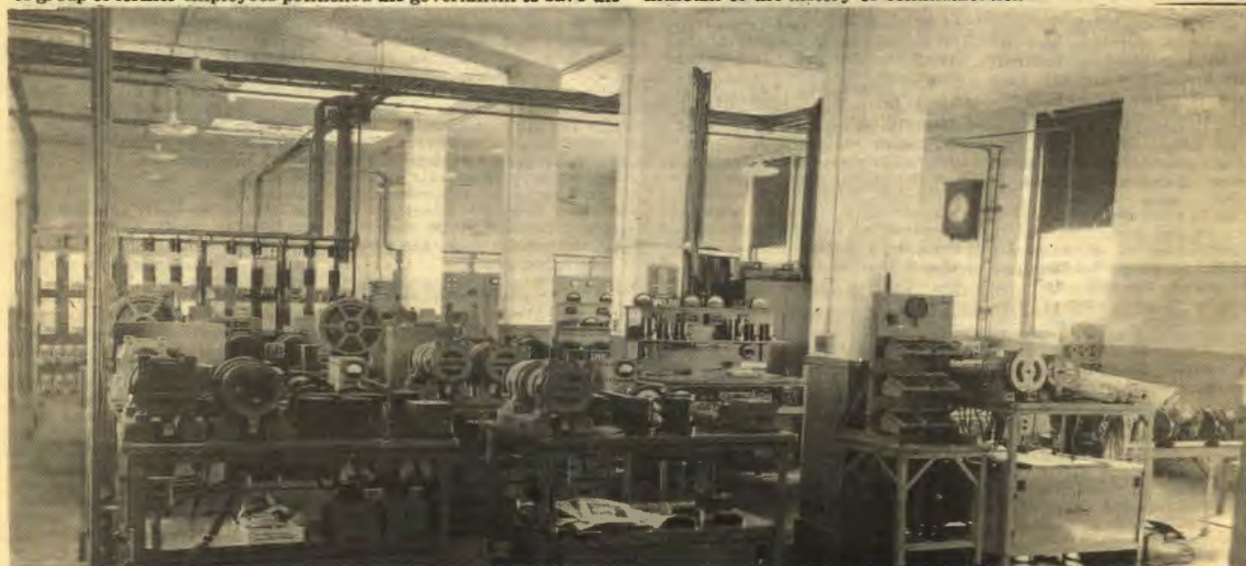
Interior view of the equipment room which is preserved much as it was when the cable station was in full operation. (Photo courtesy of the Historic Resources Division, Dept. of Tourism.)
