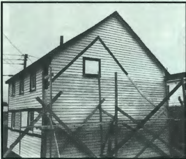
Lane House under restoration
