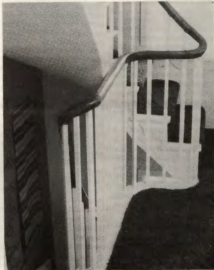
Second Floor Staircase after Rehabilitation.
