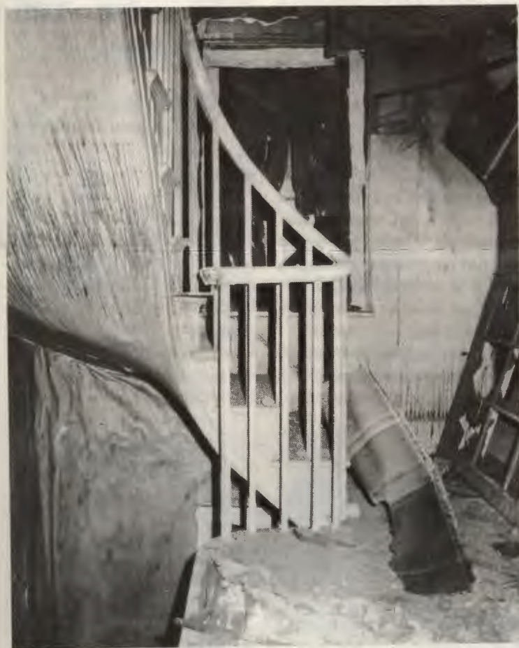
Second Floor Staircase before Rehabilitation.
