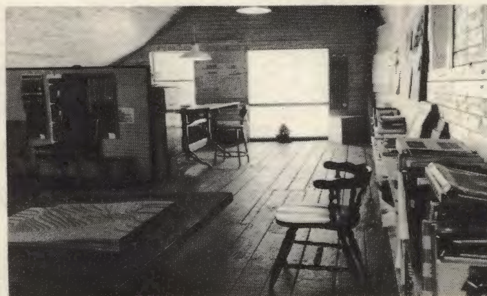
Interior view of 31 Plymouth Road, converted from warehouse to offices for architects Beaton Sheppard and Philip Pratt. Varnished tongue and groove makes a functional attractive and inexpensive finish for ceilings and walls. The original wide pine plank floor remains, improved by scrubbing and a coat of shellac. Photo Philip Pratt.
