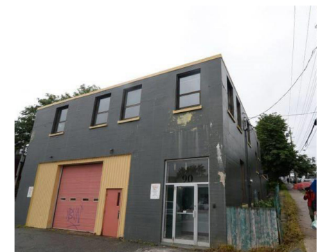
90 Duckworth Street before renovation.
