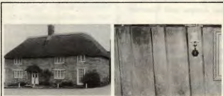
A typical three room cross-passage plan house with a central chimney in Chideok, Dorset. This three room plan was one of the common house-types built in the West Country during the early phases of Newfoundland migration.
