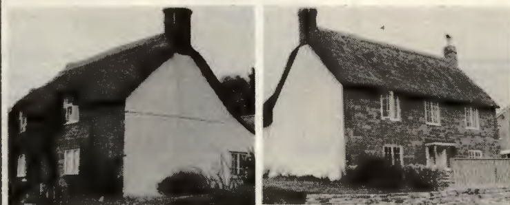
A two room central hallway plan in Chideok, Dorset, with an outshut across the back of the house. Such outshuts are common in the West Country and may provide one explanation for the origin of the Newfoundland linhay.
